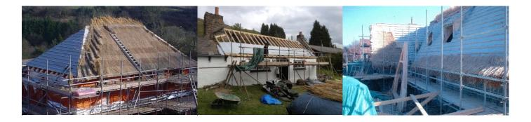
Thatch Flexi is manufactured in the UK to the specifications as recommended by Building Control. This product provides one hour fire barrier (B.S. 476: Part 3 2004) Classification EXT.S.AA. Fixed between the thatch and roof construction. In the event of a thatch fire, the thatch is sacrificial and untreated. The Thatch Flexi is a lightweight glass fibre fabric coated both sides with a polyurethane polymer containing micronised aluminium.
